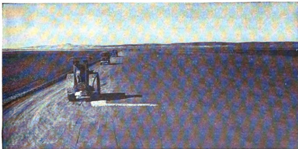
③ Compacting with roller and trucks: Note corner marker of white stone rolled into surface.
